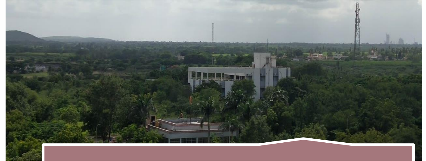
Dense plantation behind Admin Building
