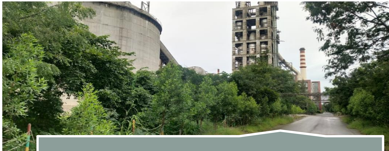
CCR Building Area
